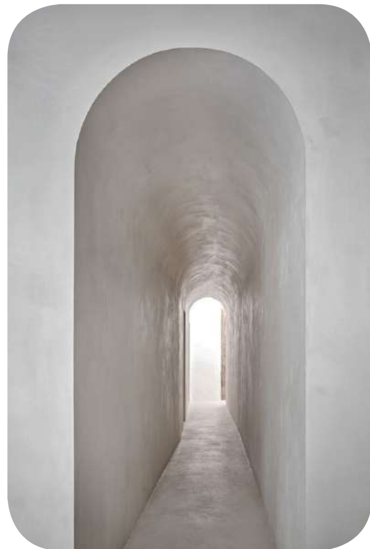
Venetian Plaster to curve blade wall
