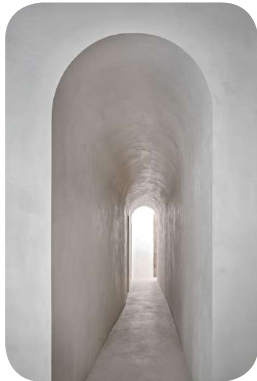
Venetian Plaster to curve blade wall
